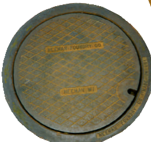
Figure 4 Black oxide begins forming. Approximately 1 to 2 months.
